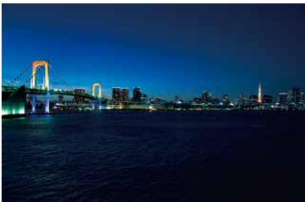
Rainbow Bridge in Odaiba © Bureau of Port and Harbor, TMG
